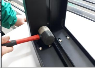
**Step 20:** Place this profile in the frame, on the vertical side, on the opposite side of the handle (the back of the sash);
