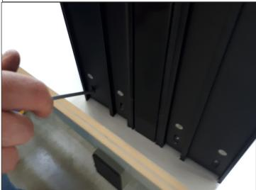
**Step 9:** After aligning the corner tighten (but not to the maximum) the screw of an outside corner bracket;
