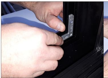
**Step 13:** Place the aligning corner brackets in their designed place on the inside of the frame;
