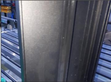
**Step 22:** This profile must be mounted where the sashes close on the frame, and must be binded with screws in the already existing holes of the frame and of the profile.
