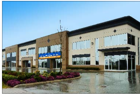
DOOR DIVISION & PREHANGING FACILITY
