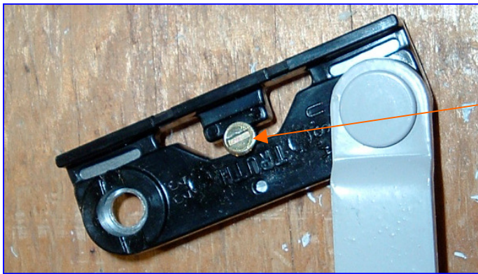
Set screws. Located at sides of vent on hinge arm.
